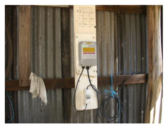
At this stage of the installation, the wiring has not been secured. [A wet day job].
