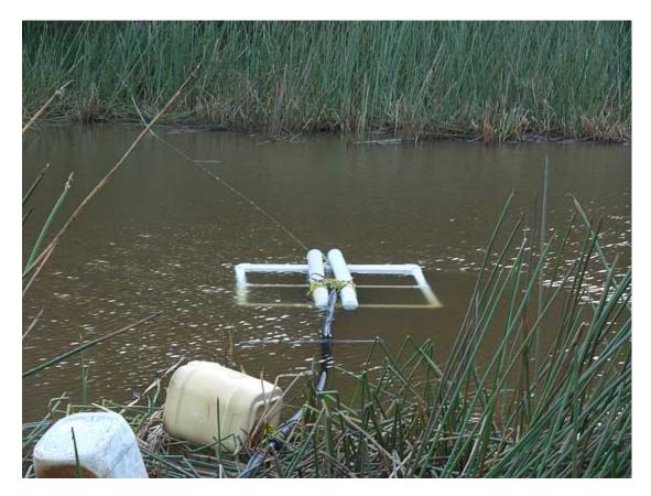
The plastic empty containers are tied to the delivery pipe to keep it more or less horizontal over 20M from float to the shed. Close inspection shows the power cable tied to the delivery pipe. The white cord running across the dam was/is used to keep the float positioned over the deep water and straight out from the shed [behind camera].
