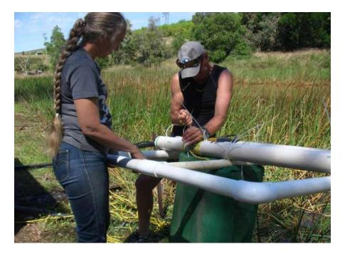
Wendy and Richard added additional floatation tubes to the top of the "in-dam assembly" before our second attempt to launch the suction assembly across the Cumbungi fringe of the dam. The additional hard poly floatation pipes also have the pump's delivery pipe [inch and a quarter soft-poly] tied to them to reinforce the delivery pipe.
