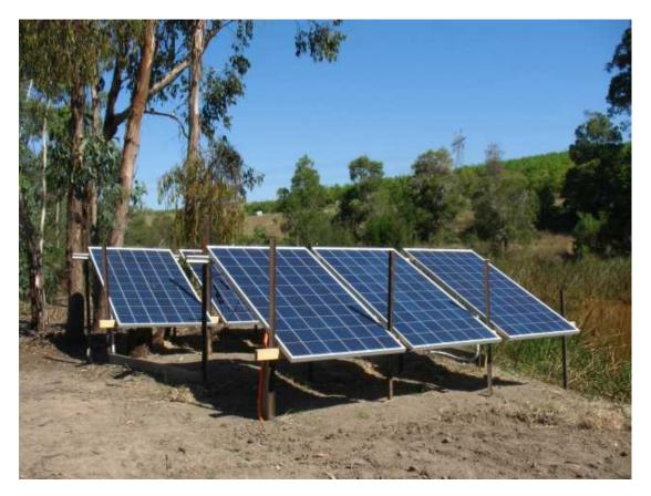
Solar arrays working. Note orange conduit to connect to control panel in pump shed.
