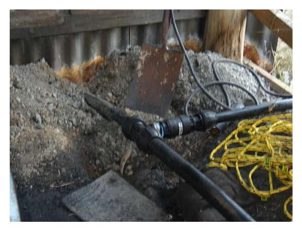
This connection causes the water to go up the hill. There is a non-return valve on the solar pump delivery line going out of the shed to the right, so that the pump does not have to push all the water in the long pipe upon start-up and the water in the long pipe "up the hill" will not run back into the supply dam via the solar pump.
